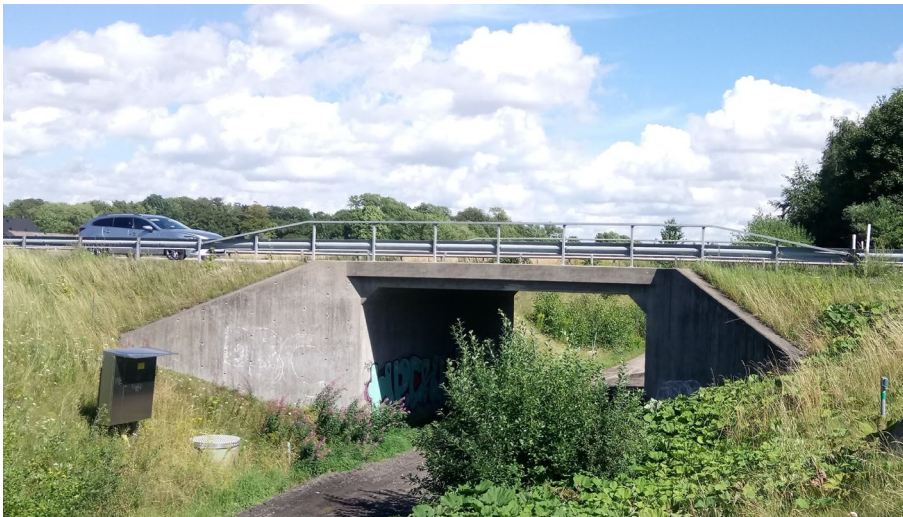
Fig. 2.1. A portal frame bridge.
